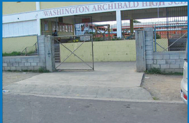
■ MAIN ENTRANCE GATE
