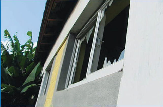
■ WINDOWS AT TOILET BLOCK
