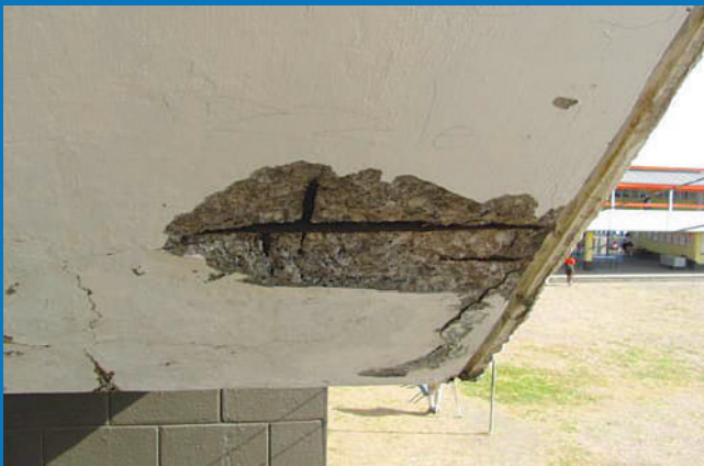
■ SPALLING CONCRETE
