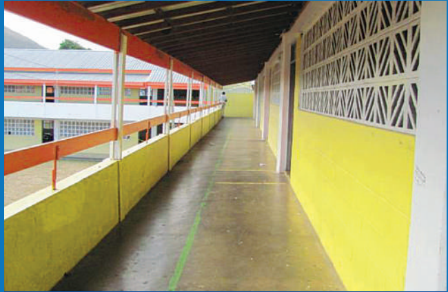
■ VENT BLOCKS - NO WINDOWS
