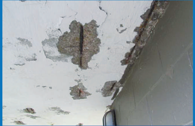
■ SPALLING CONCRETE
