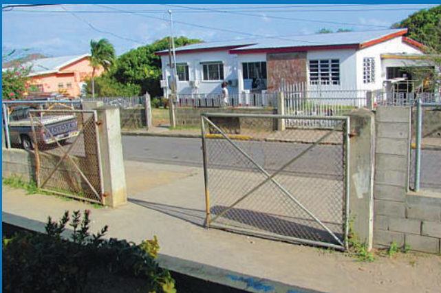
■ MAIN ENTRANCE GATE
