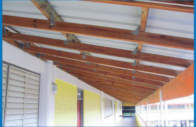
■ HURRICANE STRAPS IN OPEN ROOF
