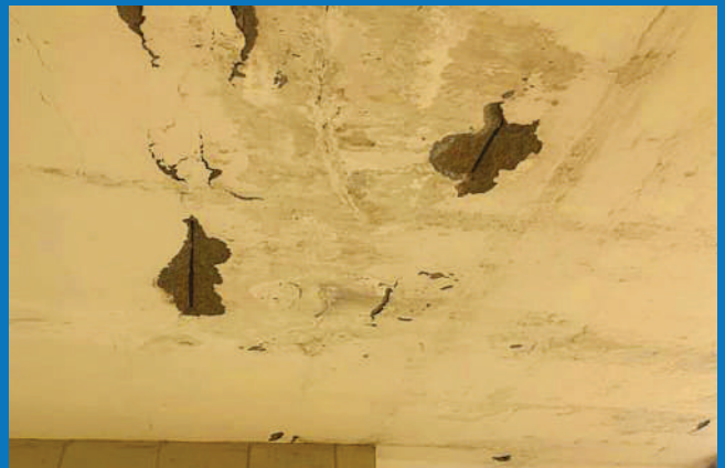
■ SPALLING CONCRETE
