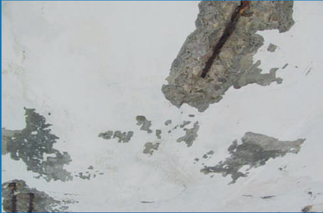
■ SPALLING CONCRETE
