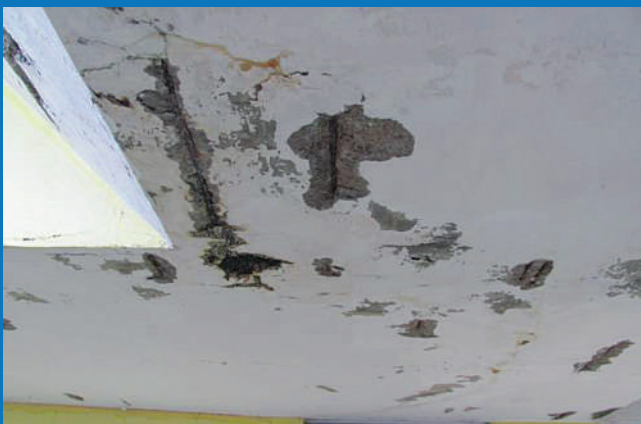
■ SPALLING CONCRETE
