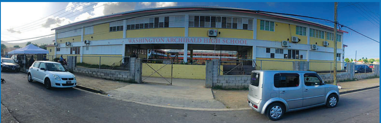
■ MAIN ENTRANCE GATE
