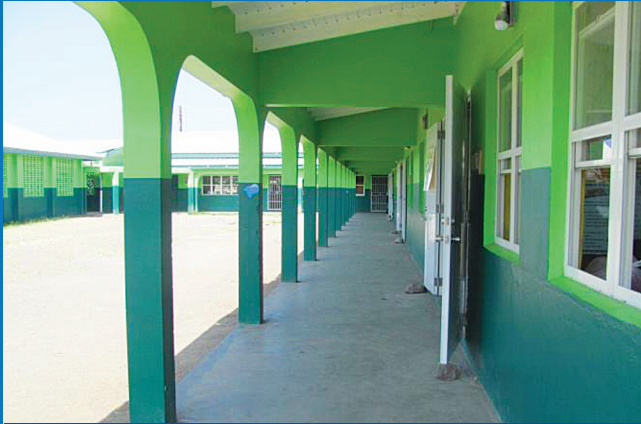
■ REINFORCED CONCRETE COLUMNS AND BEAMS SUPPORTING LIGHTWEIGHT TIMBER ROOF STRUCTURE
