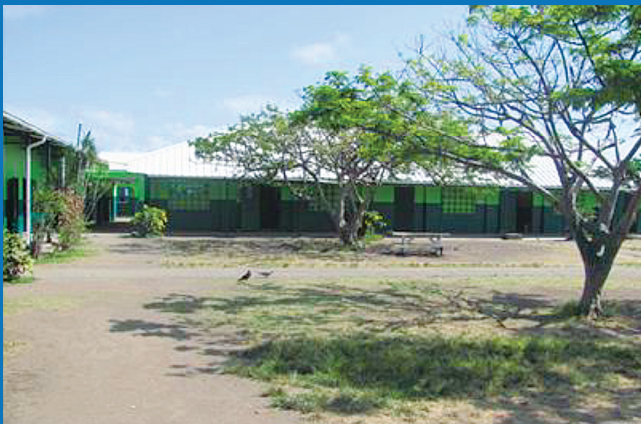
■ GATHERING / ASSEMBLY SPACE FLOODS IN HEAVY DOWNPOURS
