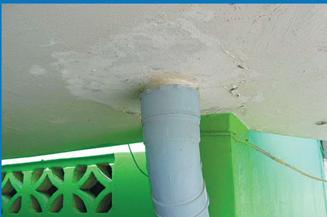
■ RECENT REPAIRS TO ROOF DRAIN
