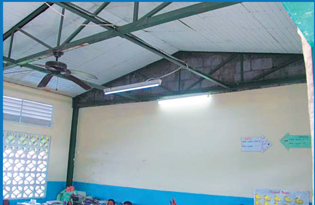
■ STEEL TRUSSES WITH TIMBER FALSE CEILING
