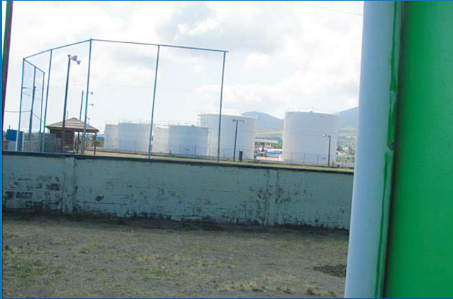
■ PETROLEUM STORAGE FACILITY ADJACENT TO SCHOOL
