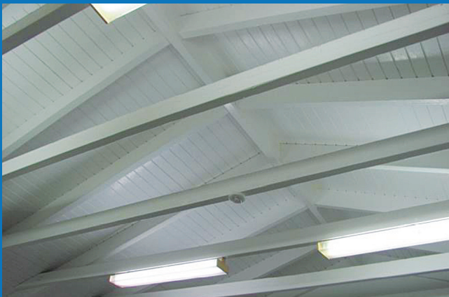
■ LIGHTING IN NEW BLOCK APPEARS ADEQUATE
