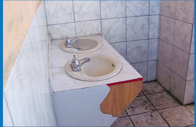
■ INTERIOR VIEW - TOILET BLOCK
