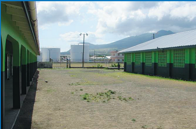
■ PETROLEUM STORAGE FACILITY ADJACENT TO SCHOOL
