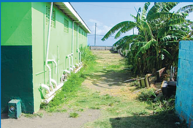
■ EXTERIOR VIEW - TOILET BLOCK
