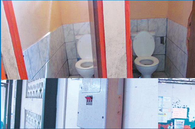
■ INTERIOR VIEW - TOILET BLOCK
