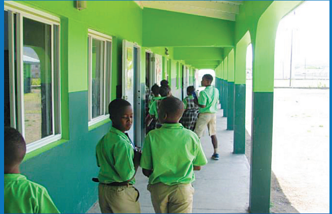
■ REINFORCED CONCRETE COLUMNS AND BEAMS SUPPORTING LIGHTWEIGHT TIMBER ROOF STRUCTURE
