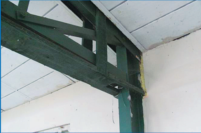
■ STEEL TRUSSES WITH TIMBER FALSE CEILING
