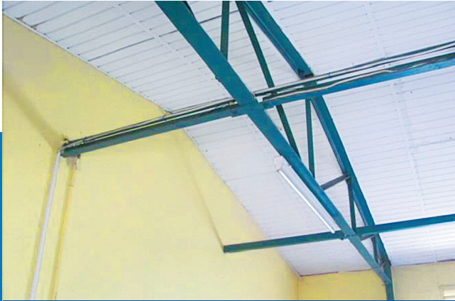
■ STEEL TRUSSES WITH TIMBER FALSE CEILING
