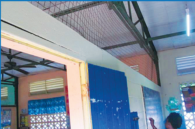
■ STEEL TRUSSES WITH TIMBER FALSE CEILING
