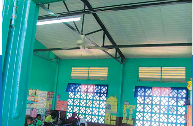
■ STEEL TRUSSES WITH TIMBER FALSE CEILING
