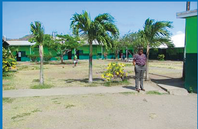
■ GATHERING / ASSEMBLY SPACE FLOODS IN HEAVY DOWNPOURS
