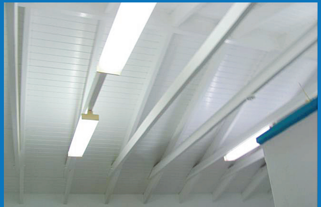
■ LIGHTING IN NEW BLOCK APPEARS ADEQUATE
