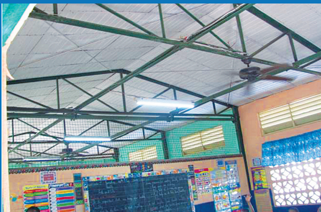
■ STEEL TRUSSES WITH TIMBER FALSE CEILING
