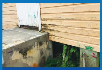
WATER-DAMAGED TIMBER STRUCTURE
