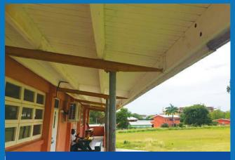
ALUZINC SHEET ROOF COVERING ON STRUCTURAL STEEL AND TIMBER COMPOSITE ROOF STRUCTURE
