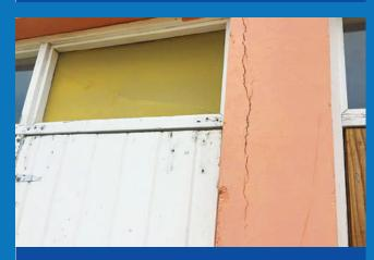
VERTICAL CRACKS IN COLUMNS
