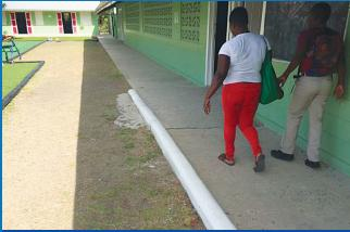
CURB WALL ERECTED TO MITIGATE FLOODING-RELATED PROBLEMS
