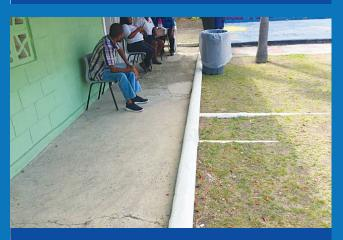
■ CURB WALL ERECTED TO MITIGATE FLOODING-RELATED PROBLEMS
