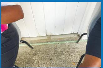
■ CURB WALL ERECTED TO MITIGATE FLOODING-RELATED PROBLEMS
