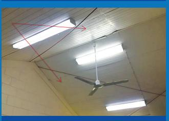
DIAGONAL BRACING TO STRUCTURAL STEEL ROOF STRUCTURE
