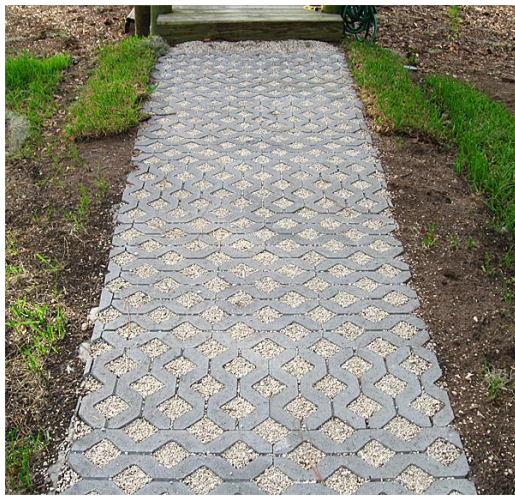
Figure 5: Installed Permeable Pavers
