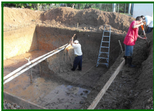
Digging of foundation for casting of footings for repeater tower.
