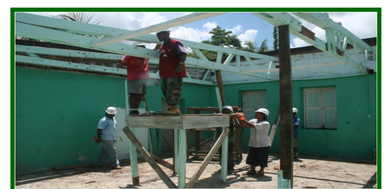
Work-in-progress on Rancho Dolores hurricane shelter.
