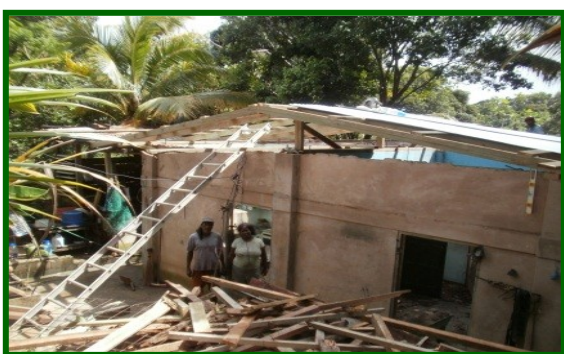
Work-in-progress on a house in the Cumana community.
