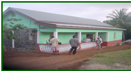
RC/MJ Renovated Community Centre.
