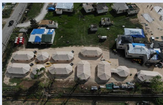
Figure 4: An aerial view of the field hospital from the Barbados Defence Force being assembled
