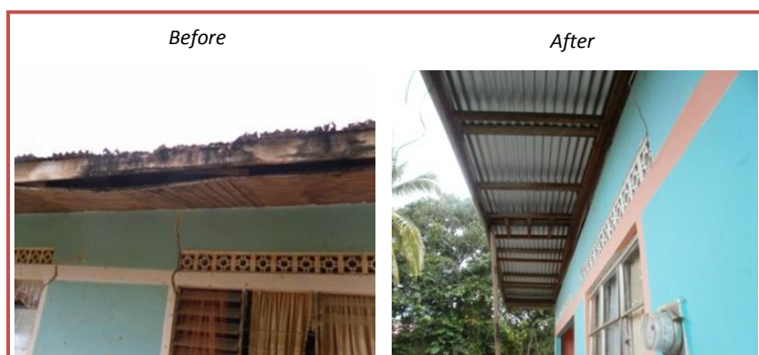
Figure 1: Roof repairs – Project C.A.R.E.
