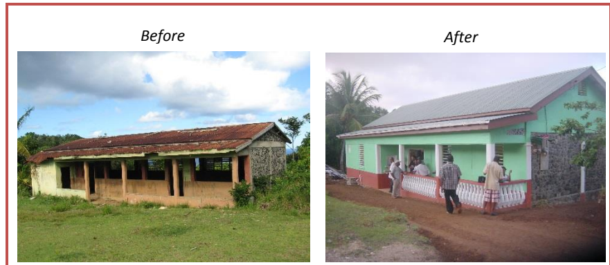
Figure 1: Before and after pictures of the Riviere Cyrique hurricane shelter
