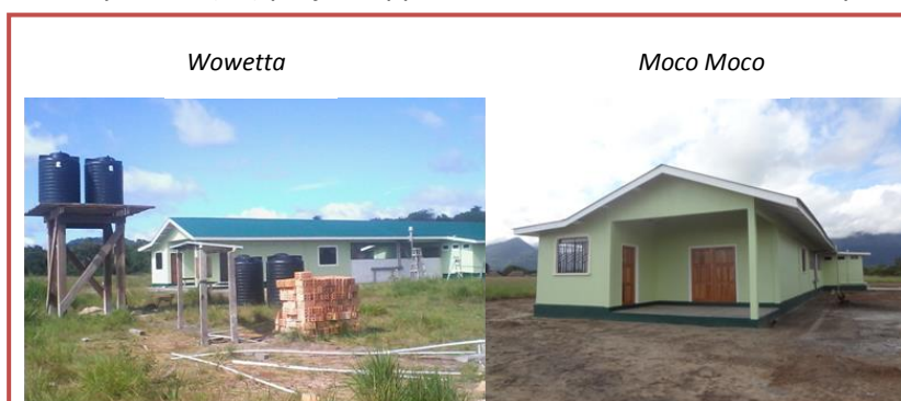
Figure 1: Farine processing and storage facilities, WVC and KMCRG projects
