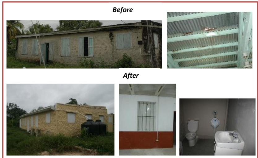
Figure 1 Renovation of the Rancho Dolores Shelter
