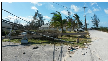
Broken poles found within assesses communities in New Providence
