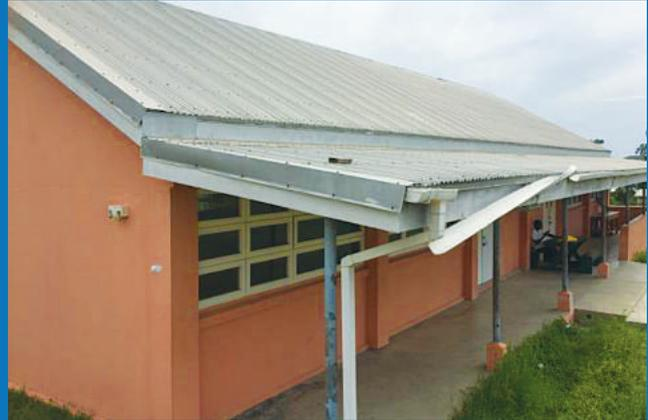
■ ALUZINC SHEET ROOF COVERING ON STRUCTURAL STEEL AND TIMBER COMPOSITE ROOF STRUCTURE
