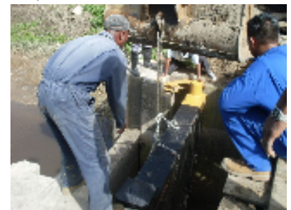
Newly fabricated sluice (flood) gate being installed.
